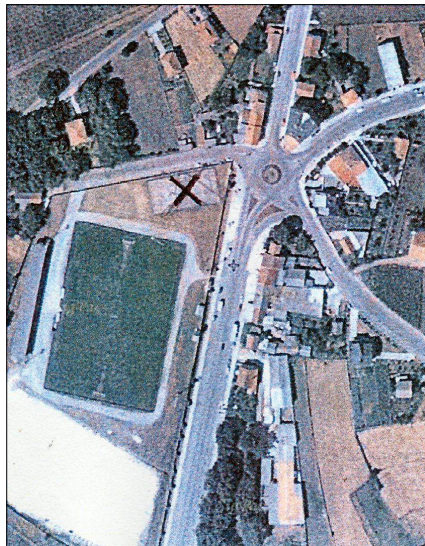
Fig. 1. Aerial view of the site of the sundial building at Lalín.
